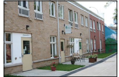
St. Lawrence Street Apartments Toronto, Ontario
